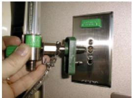
particular orientation is critical to the design, avoid symmetry. For example, use nonsymmetrical hole patterns.
