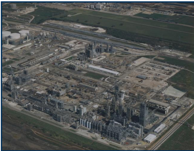
Figure 9. Phillips complex before the accident
