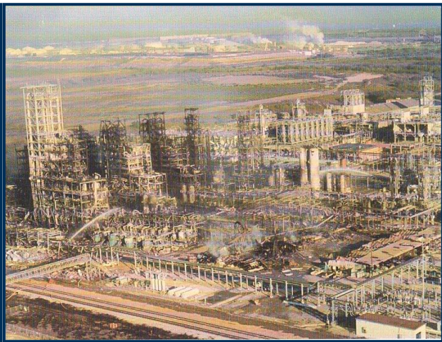
Figure 10. Phillips complex after the accident
